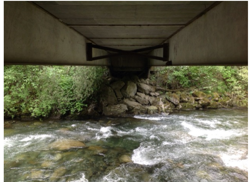
Left Bank Abutment when facing downstream
