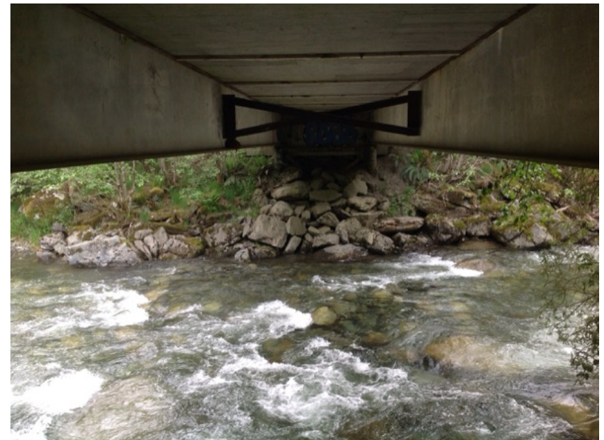
Right Bank Abutment when facing downstream
